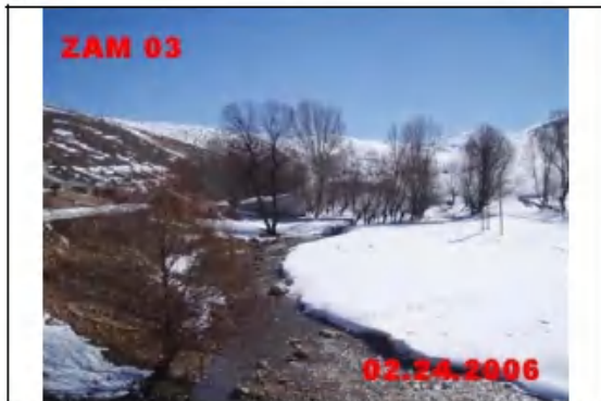
Pipe line crossing the river 2/24/2006
