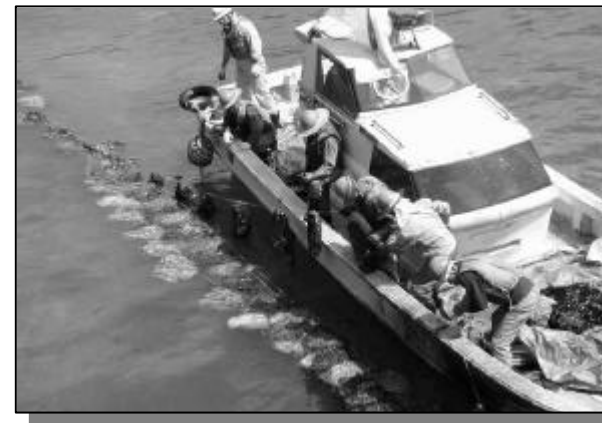
Deploying the oil snare
